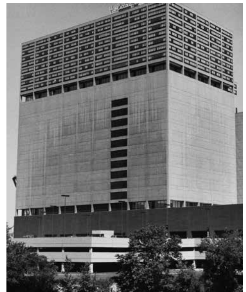
Figure 3 Water washing and dirt deposits.
